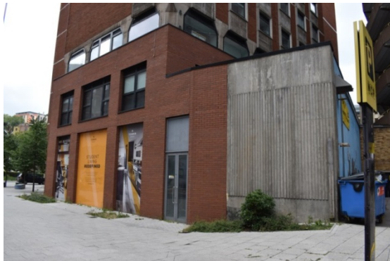
Rupert Street Car Park (P235): Here an already open bed at the base of concrete wall provides a 'quick win' opportunity for a green wall. With the addition of a simple support structure fixed to the concrete wall, climbers could be planted to provide a green/ living wall on the building elevation.
